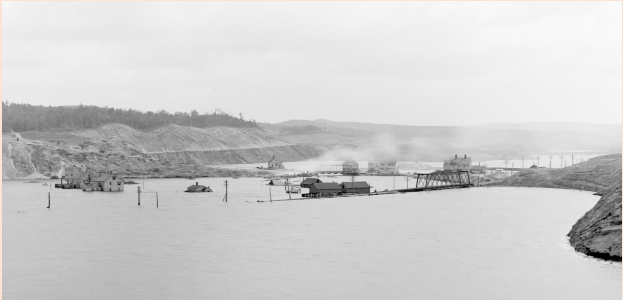
Looking south at Sawyer's Mills as seen at high water after the June 1903 deluge. These buildings were later removed before the final filling of the reservoir.
