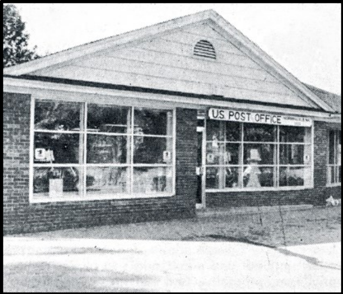
MORNINGDALE POST OFFICE 63 MAIN STREET Photograph Courtesy of Boylston Post Office
