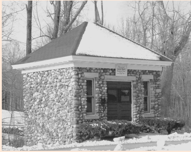
Stone Switching Station Built 1913 - Boylston Center BHSM Collection
