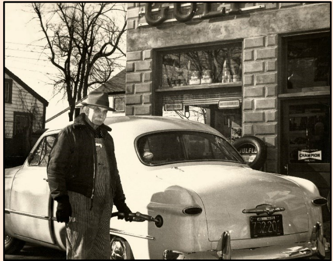
Gramps Brigham Gasoline Station, Boylston, Massachusetts BHSM Photograph Collection
