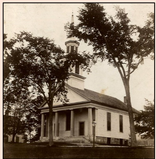
Boylston Church -Third Meeting House This steeple blew off roof in 1903 storm BHSM Photograph Collection
